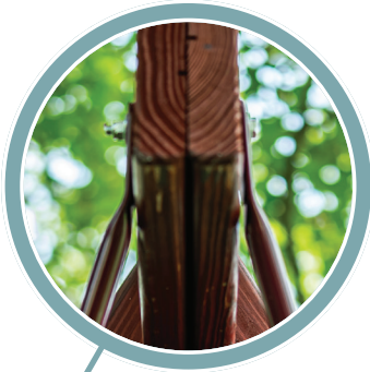
Heavy-duty, double 2x6, vertical-edge swing beams.
