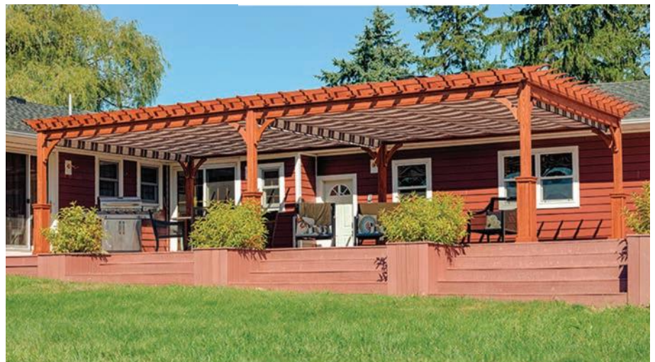
16'X32' WOOD TRADITIONAL (2) EZ Shade Canopies, Superior Posts, & Canyon Brown Stain
